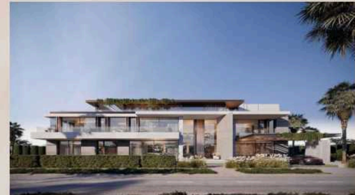
MEYDAN RACECOURSE MANSIONS Completion 2027
